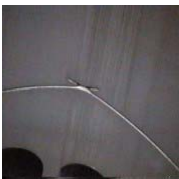
Oil grooves in a cylinder liner
