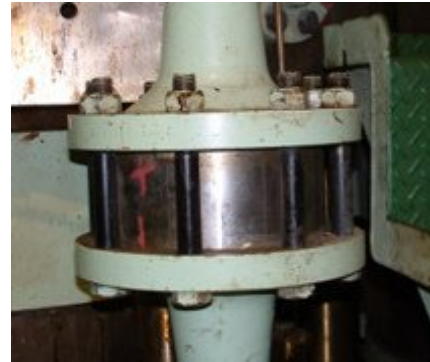
Flame Arrestor Sulzer RTA
