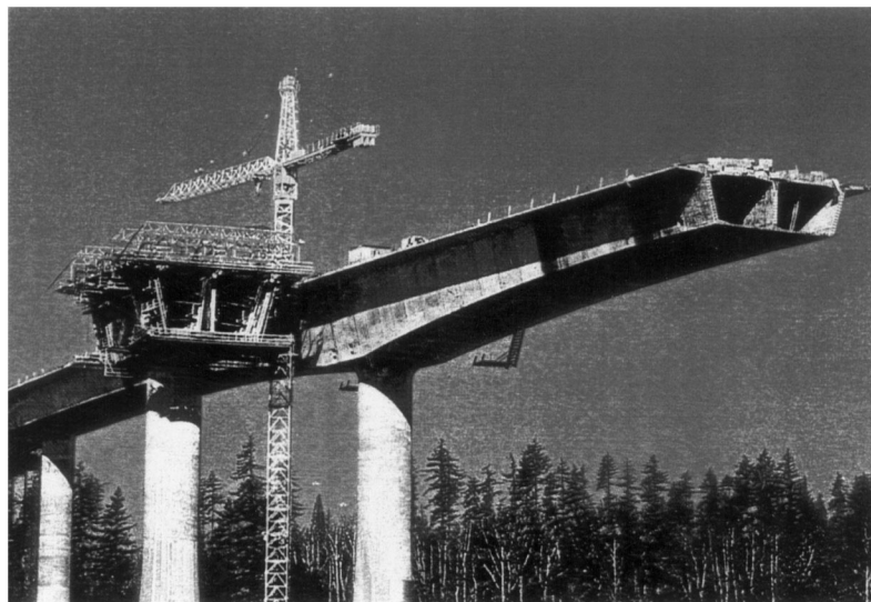
Fig. 5. Glen Jackson Bridge crossing the Columbia River in OR, USA.
