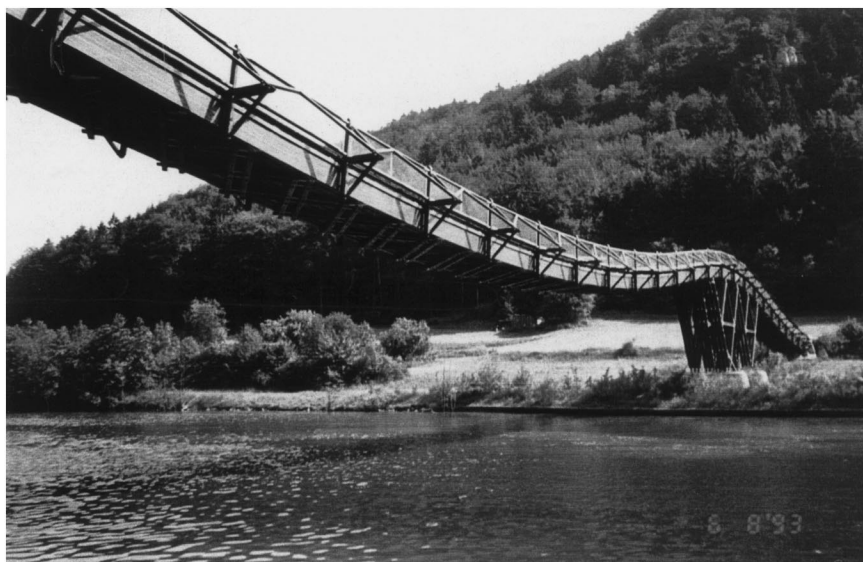
Fig. 11. A pedestrian timber ribbon bridge in Essing (Germany), span of 73 m.
