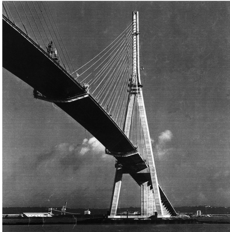
Fig. 2. Pont de Normandie over the mouth of Seine River, cable-stayed, span 856 m.
